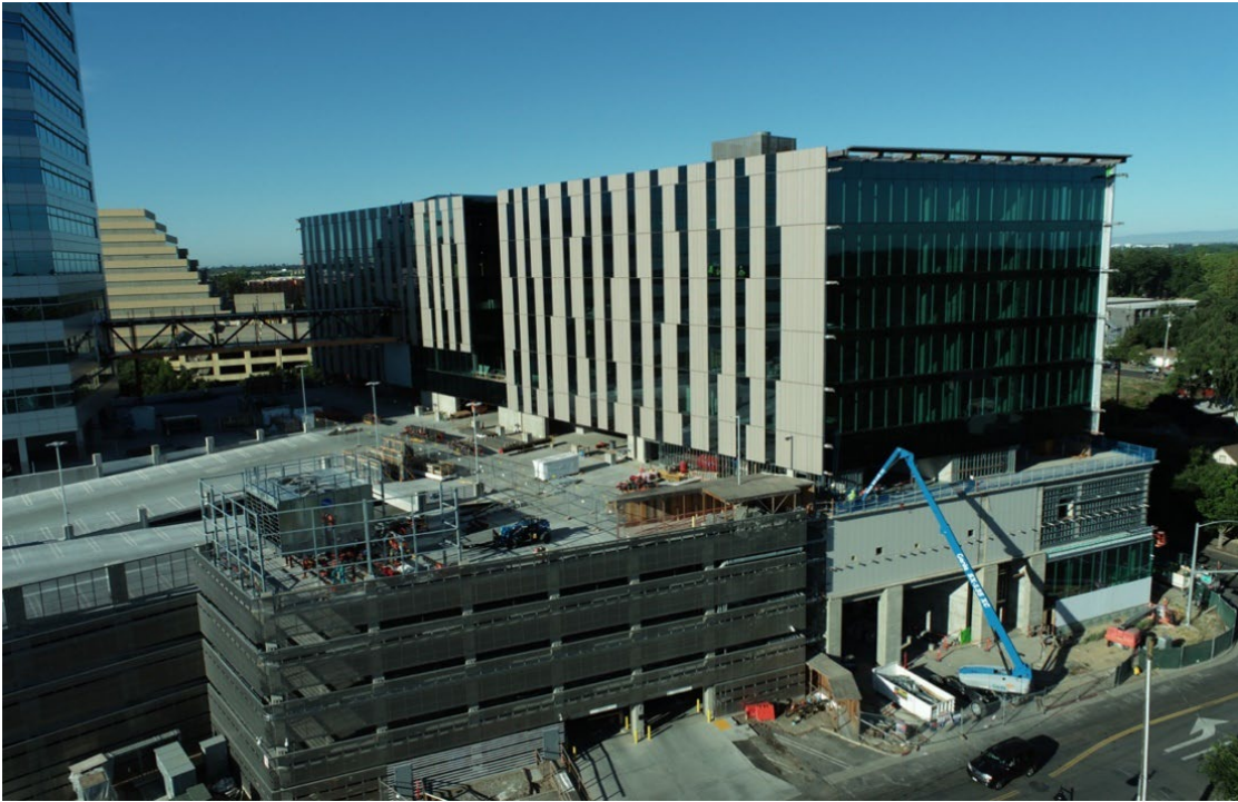
Northeast side of building
