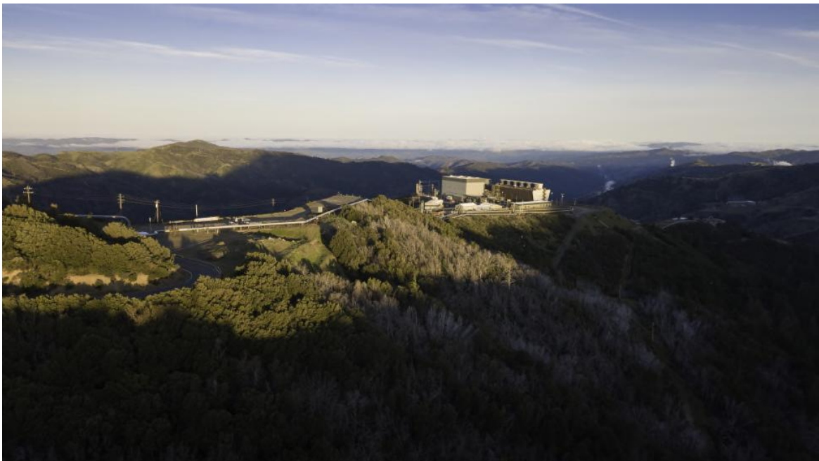
Calpine's Geysers Sonoma Unit 3 power plant at The Geysers. Photo courtesy of the © 2025 Calpine Corporation. All Rights Reserved.
