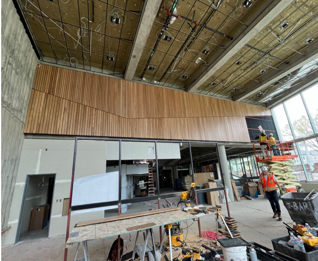
Cafe wood panel installation
