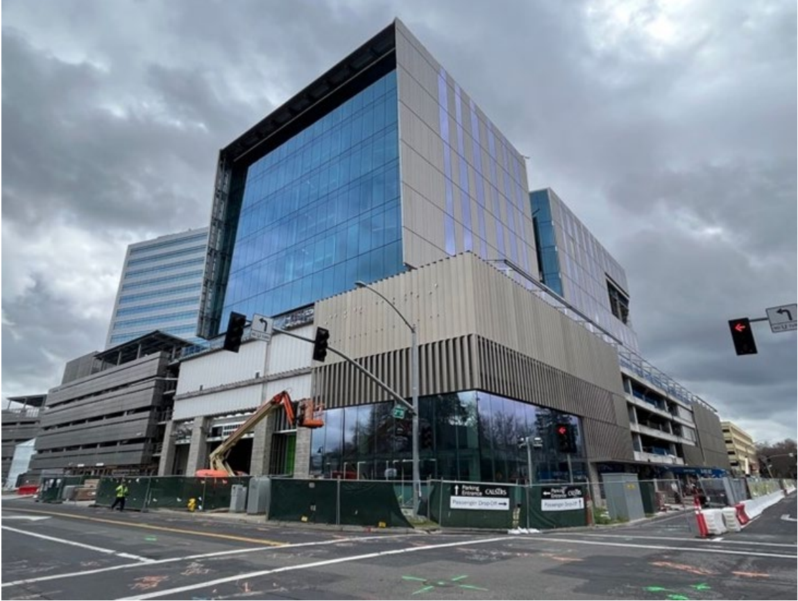
Northwest garage panel installation
