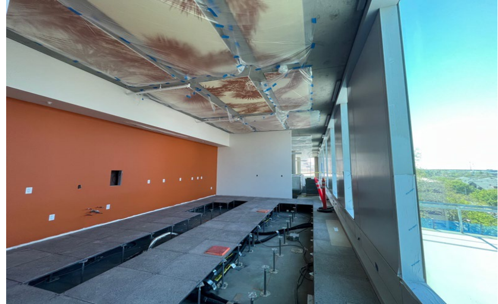
O3 south break area
