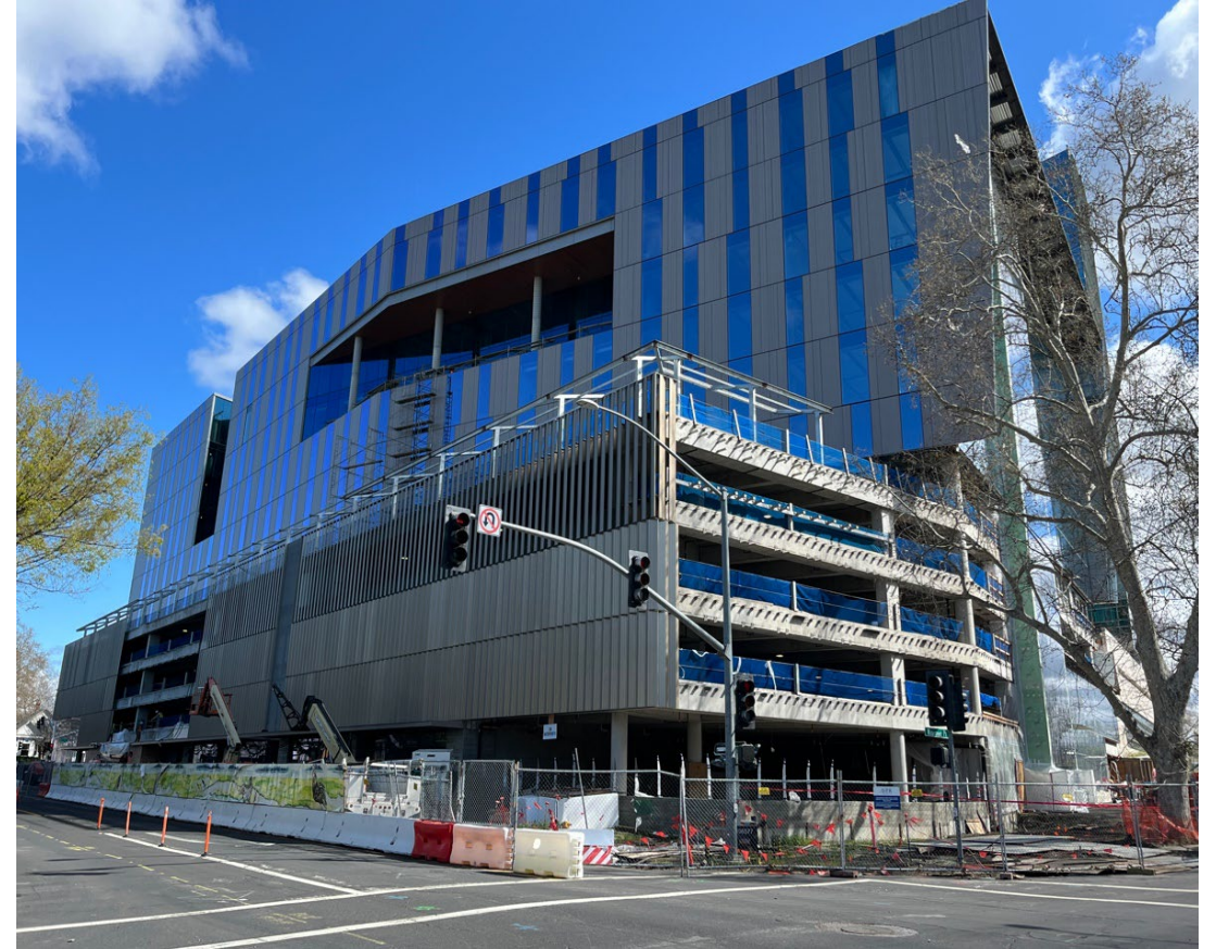
Southwest garage panel installation
