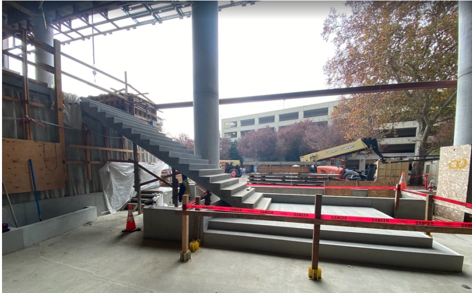
Communicating Stair Installation at Atrium Board-form Concrete
