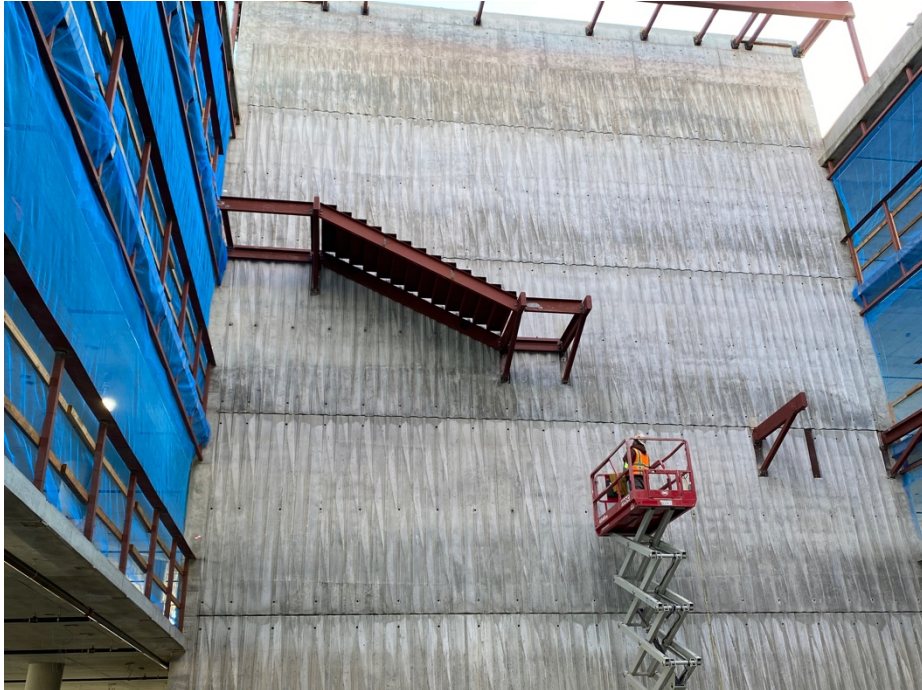
Communicating Stair Installation at Atrium Board-form Concrete
